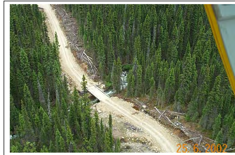
Photograph #1284. Recent bridge installation on tributary stream
